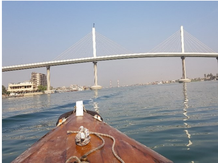
Shatt Al-Arab River Bridge (1188m), opened in 2017.
